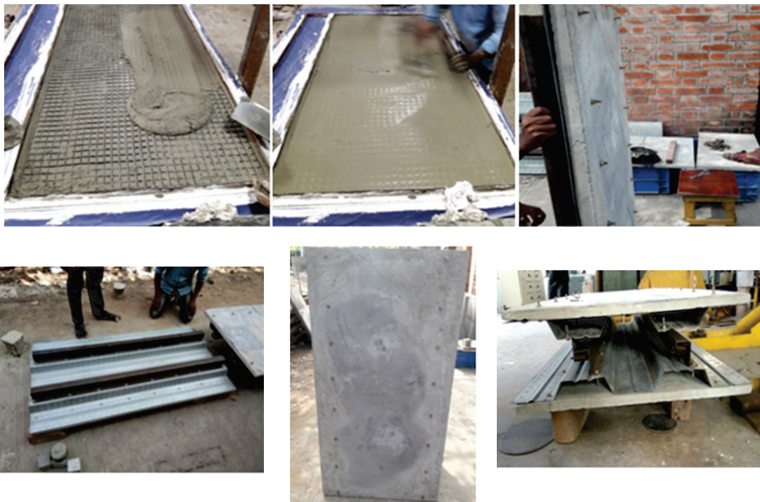
Figure 4: Various stages involved in the fabrication of TRC-cold form steel cavity wall panel system
