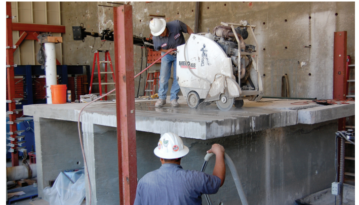
Figure 3(a): Saw being used to cut grooves for placement of the FRP strips
