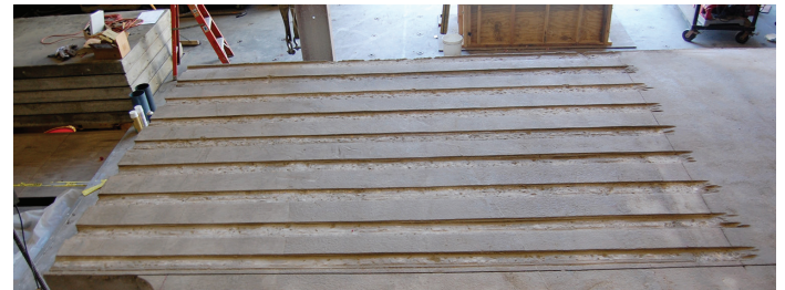
Figure 3(b): Grooves prior to placement of adhesive and FRP strips
