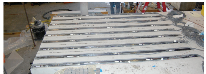
Figure 3(c): Specimen with strips installed in grooves with strain gauges
