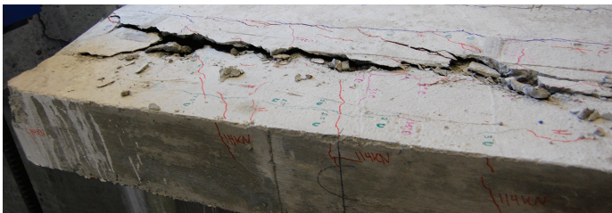
(c) Overhang edge prior to removal of loose concrete
